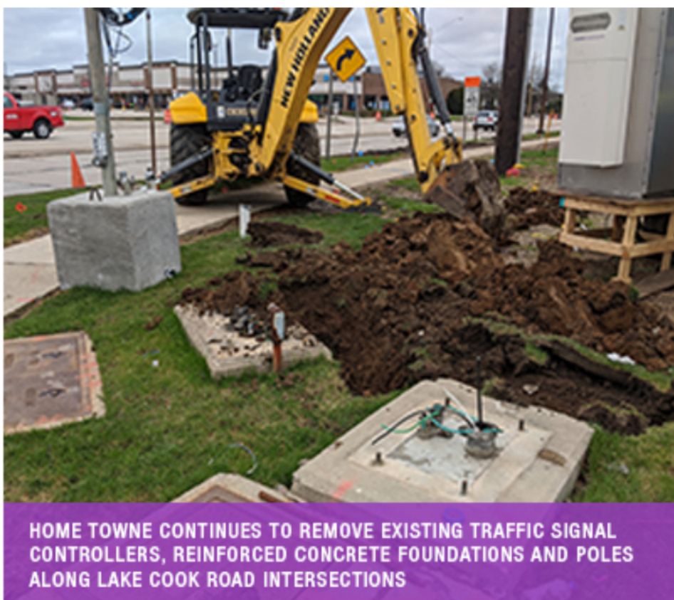
HOME TOWNE CONTINUES TO REMOVE EXISTING TRAFFIC SIGNAL CONTROLLERS, REINFORCED CONCRETE FOUNDATIONS AND POLES ALONG LAKE COOK ROAD INTERSECTIONS
